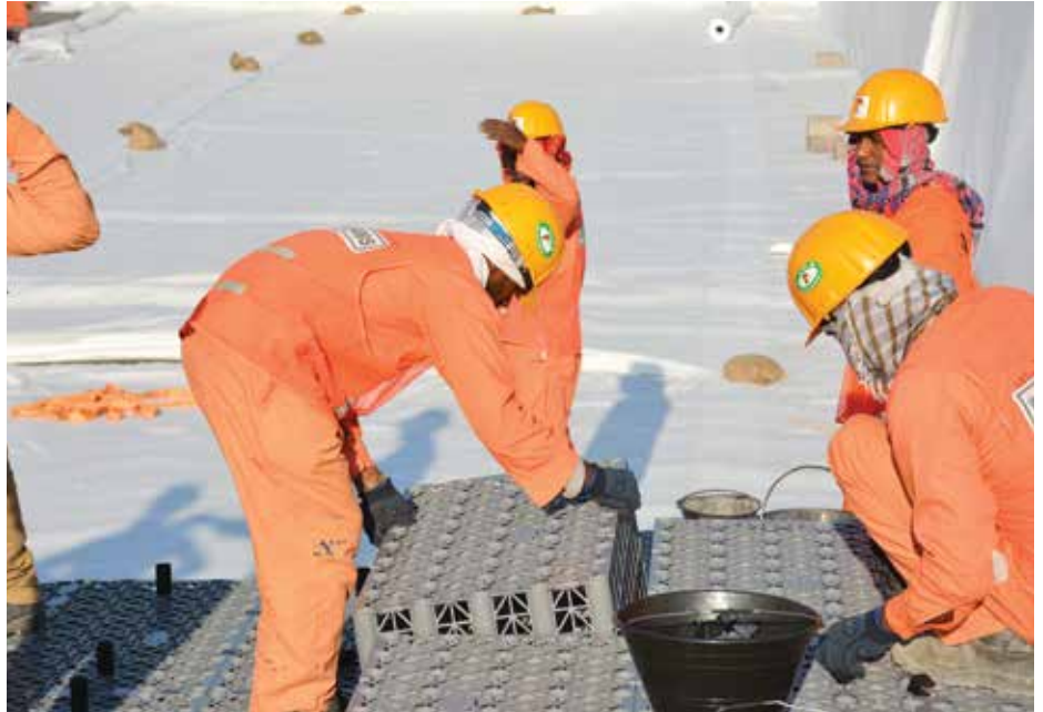
Polypipe's Polystorm geocellular water management system ... specified as a stormwater management solution at Remraam community.
